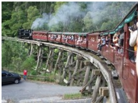
Puffing Billy Railway, Monbulk Creek bridge - note the out of gauge legs!
